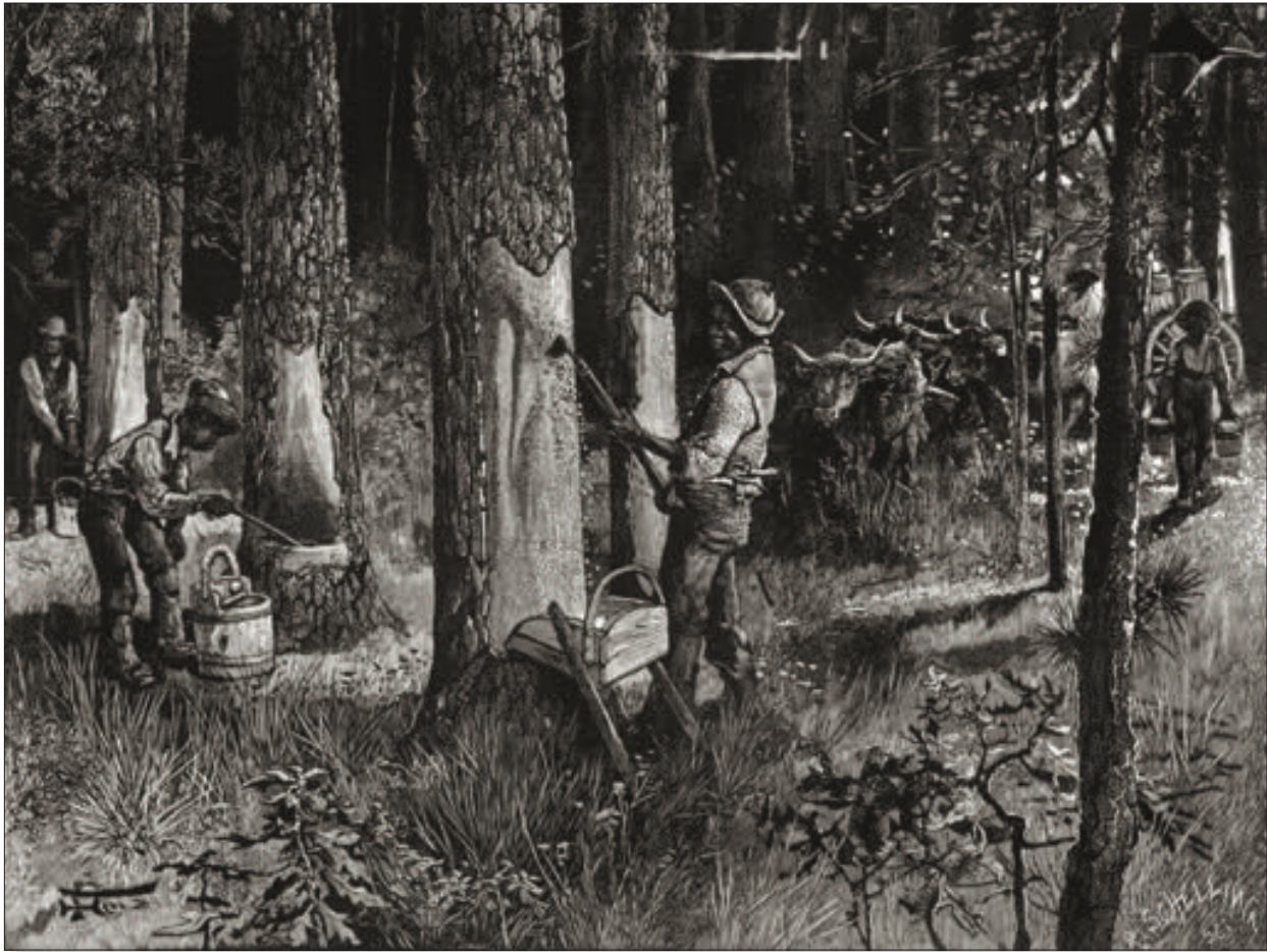
This drawing illustrates the early gum collection method. The worker on the left is dipping resin from a box cut into the base of the tree. The worker in the center is scraping the worked face to remove resin that did not drain into the box. The worker on the right is bringing a wagon with barrels to collect the resin (Earley 2004).
